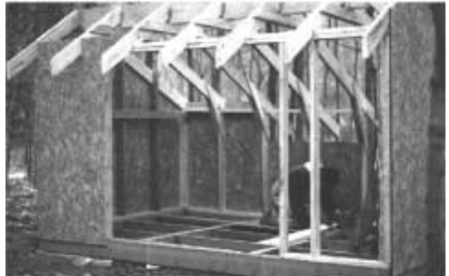
Charterhouse during the construction phase - 1990
