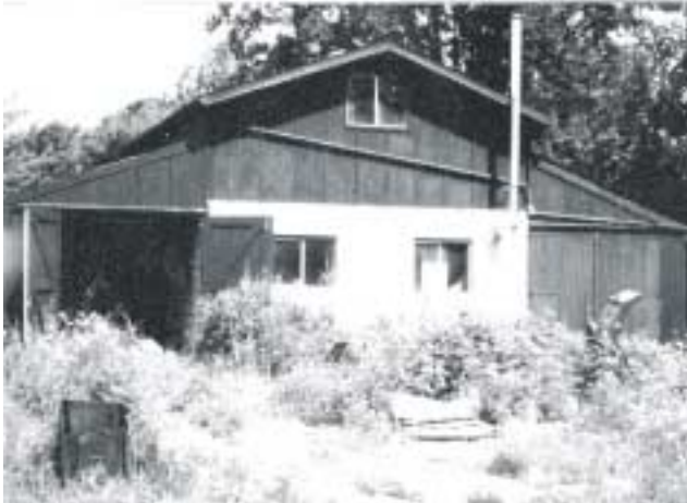
Rear of the Warden's Barn - 1993
