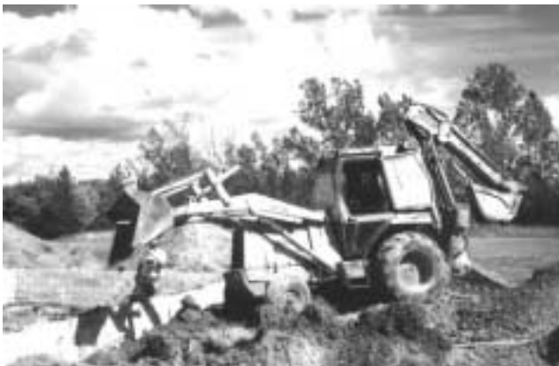
Anniversary Lodge Construction - Camp Warden Gerry Bluhm the back hoe operator- 1997
