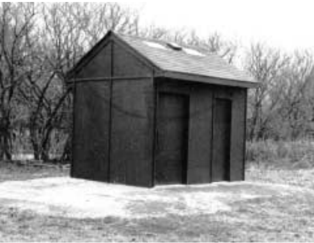
Confederation Lodge K.Y.B.O - wheelchair accessible toilet , 2 urinals and one regular toilet - 1995
